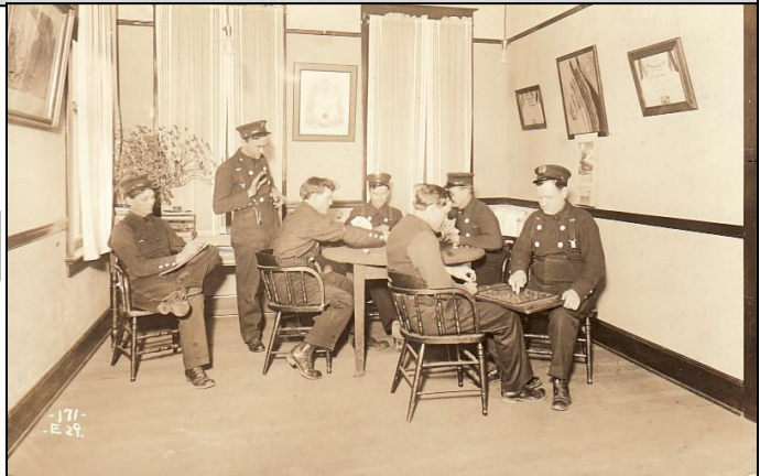
Interior of Station 29
